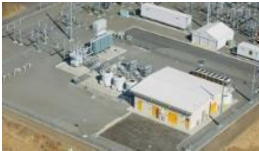
SVC PLUS (STATCOM) IGBT based
